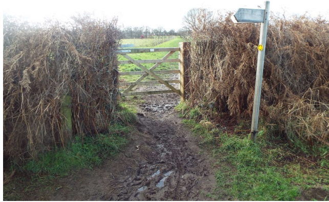
Figure 13 Easy Access Gate – Restricted by Muddy surface
