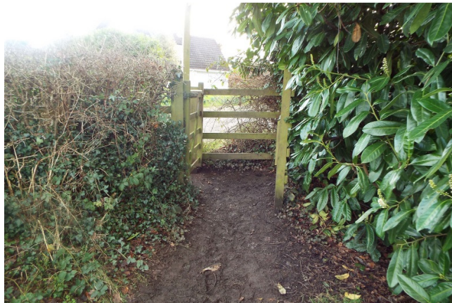
Figure 15 Footpath finishes at field gate - design restricts wheelchair access
